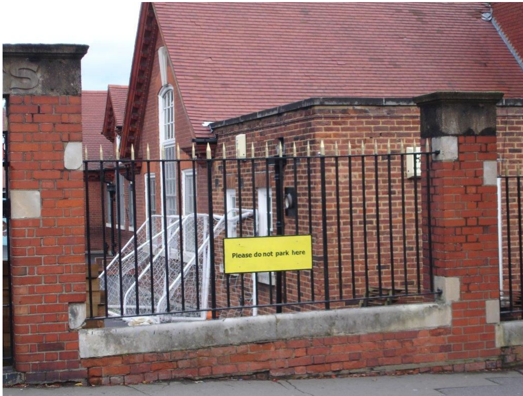
South Harringay Primary school playground before installation:
