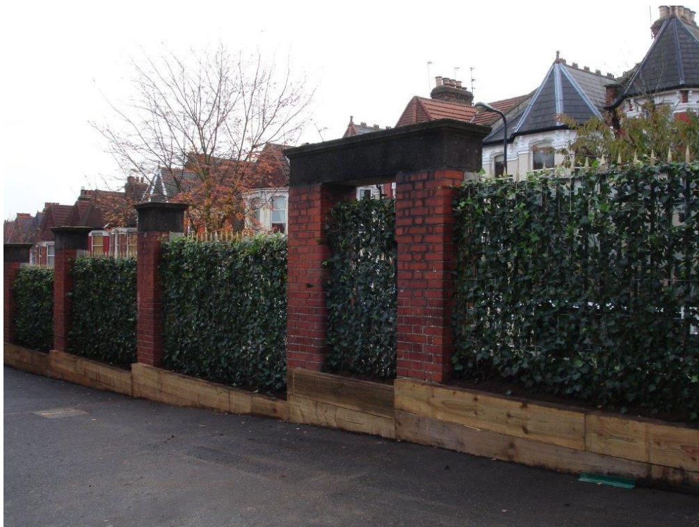
South Harringay Primary After installation
